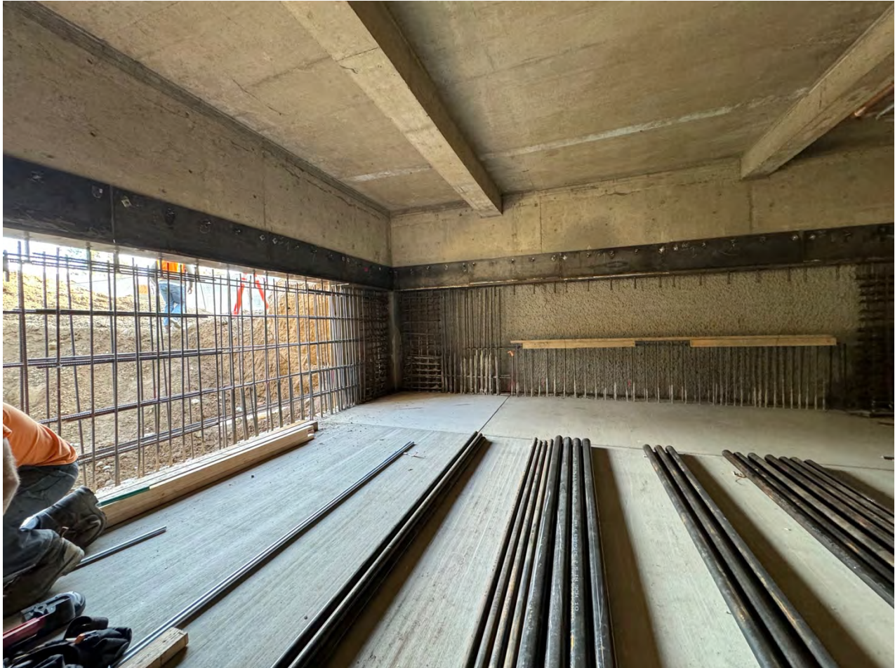
Ashland High School Humanities Building Continued Structural Reinforcement
